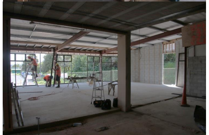
Update to ACCC Mangere Hall Renovations – Nov 8 2016
